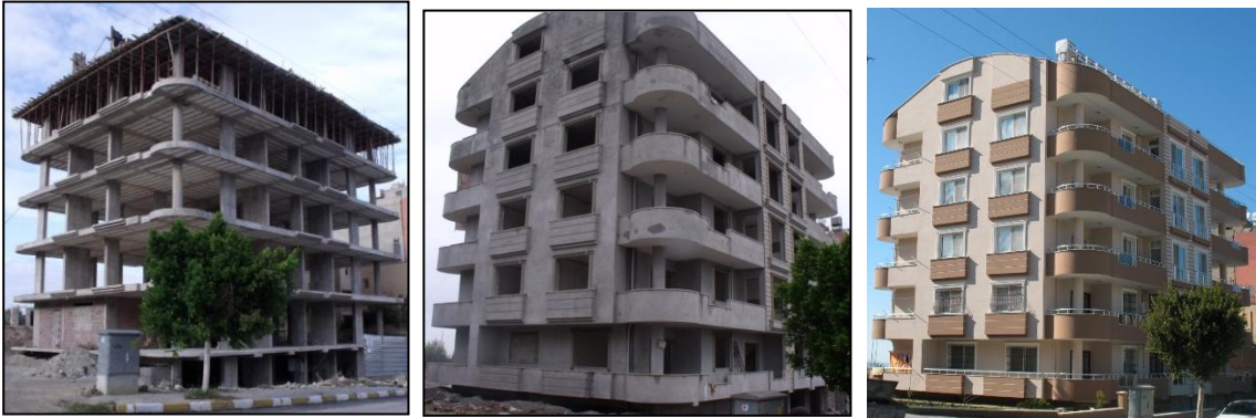
Fig. 1. without infill walls Fig. 2. with infill walls Fig. 3. under usage The recording period was around 30 minutes during each three stages and low pass filter was applied to eliminate the noise with frequencies higher than 15 Hz. Figure 5 shows a typical record and corresponding Fourier Amplitude obtained from stage one test.
